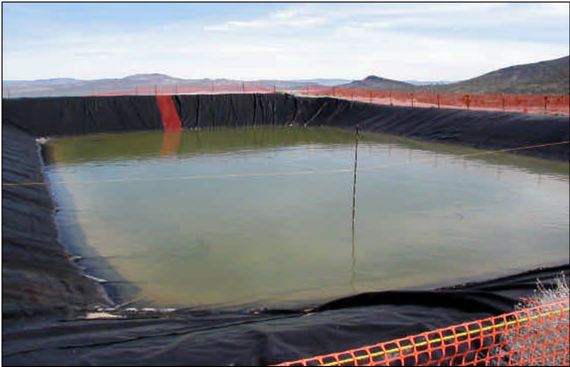
Figure 5-23. Plastic-lined Sump ER-6-2 monitored for wildlife mortality during 2005. (Photo taken by Paul Greger on December 27, 2004).
