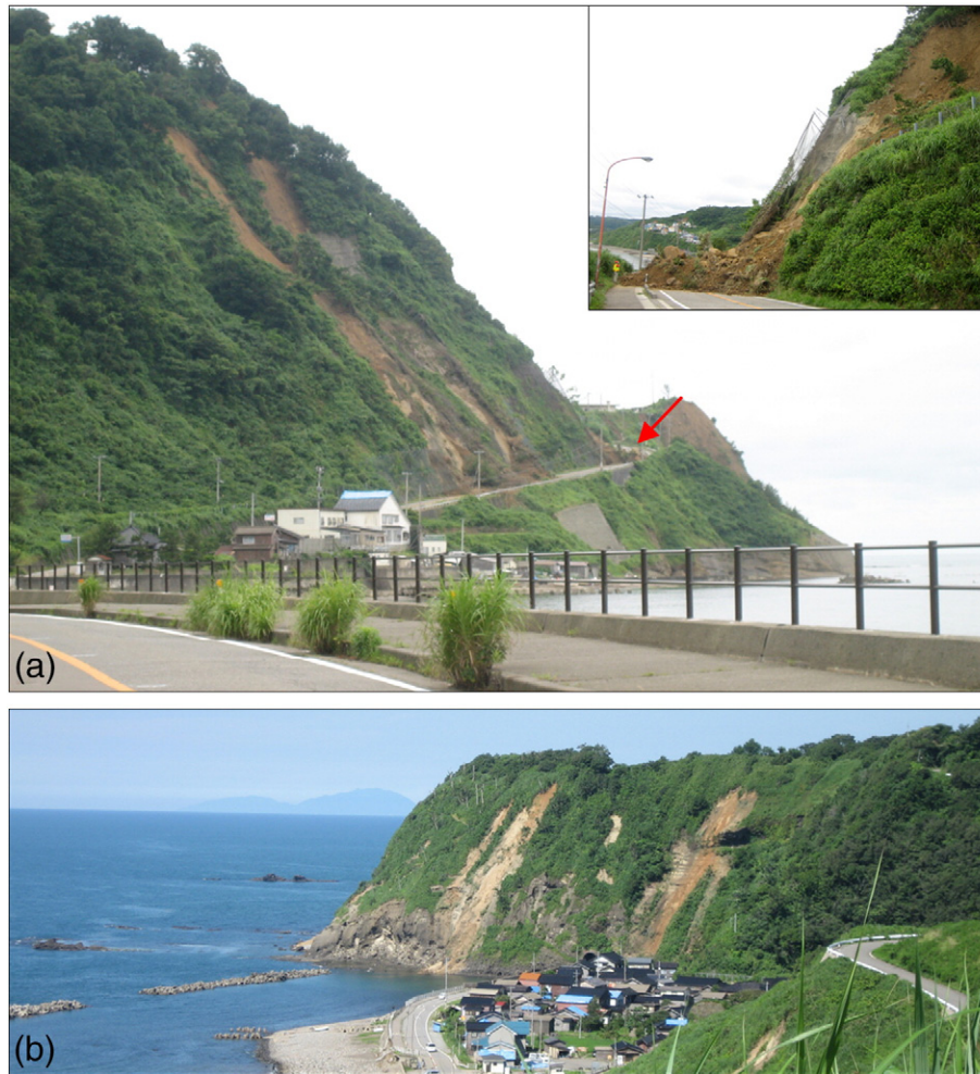
Fig. 2. Coastal landslides (a) north of Kashiwazaki at 3 km JMA epicentral distance and (b) south of Kashiwazaki at 23 km JMA epicentral distance. Arrow in (a) identifies the location of the inset image.
