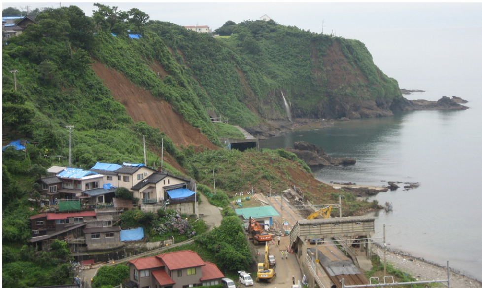
Fig. 10. The Oumigawa train station landslide located south of Kashiwazaki exemplifies the metastability and high seismic susceptibility that many coastal slopes exhibited.
