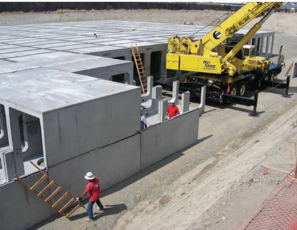
FIGURE 14 - DISCOVERY PARK INFILTRATION SYSTEM
