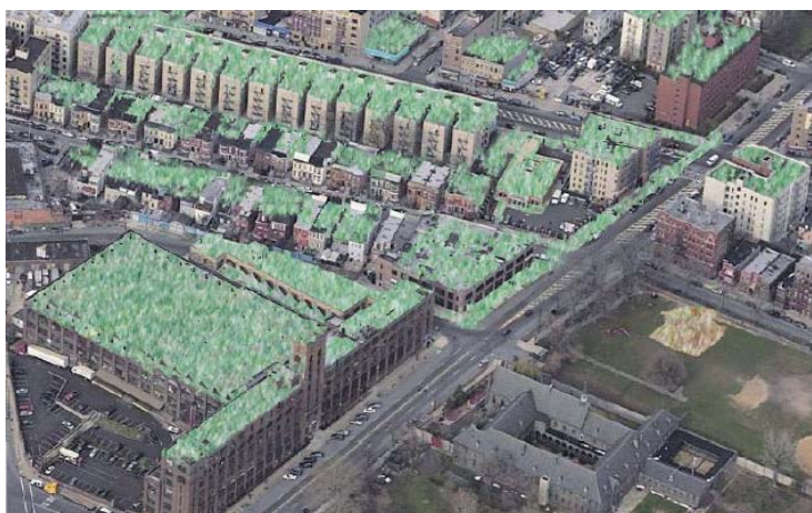
A 2006 Columbia University study performed for Sustainable South Bronx found that if 155 acres of green roofs were constructed in Hunts Point, stormwater runoff would be reduced by over 50 percent on new green spaces, capturing 1.1 million gallons of stormwater annually. The image above shows a what Lafayette Avenue would look like under this program. Image: Jin Jo (2006).
