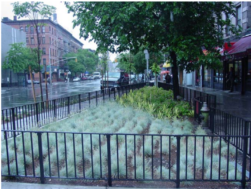
This Greenstreet at 110 th Street and Amsterdam Avenue in Manhattan was designed to capture surrounding stormwater. The formerly paved site now provides substantial community benefits. Design by Jeff Kieter, NYC Parks Department.
