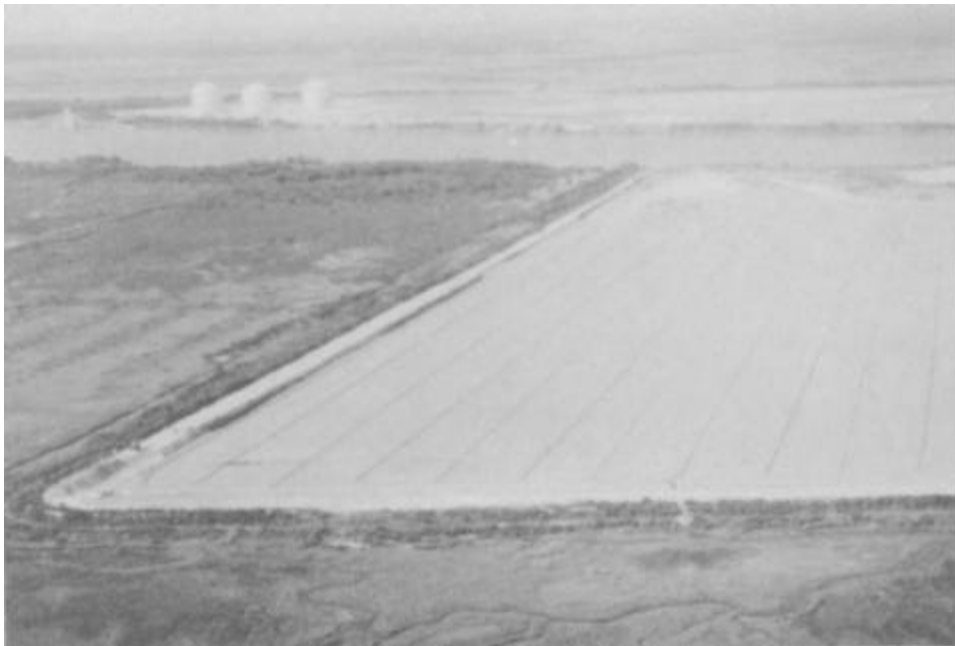
Figure 5-22. General view of confined disposal area showing parallel trenches in place
