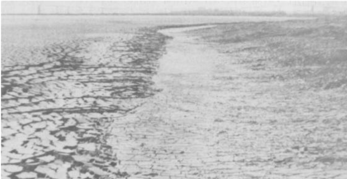
Figure 5-9. Shallow initial perimeter trench constructed by dragline operating from perimeter dike
