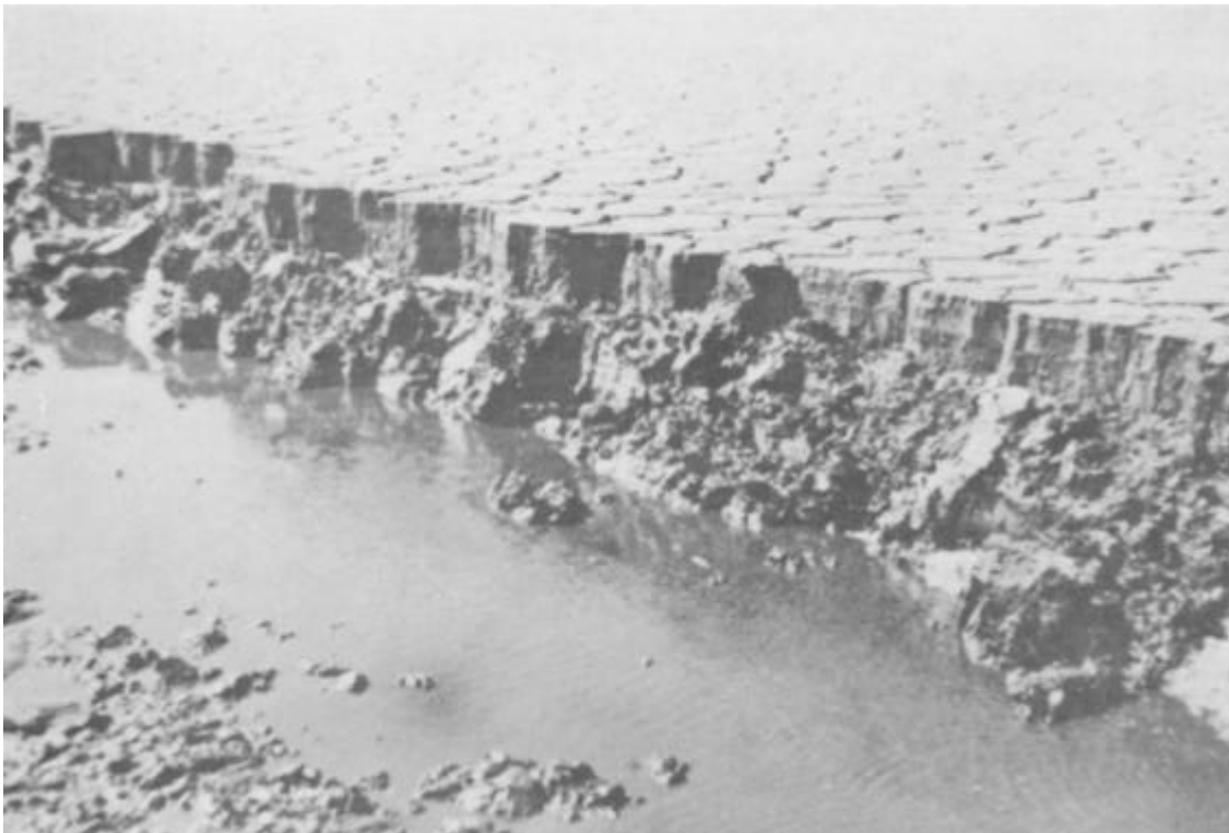
Figure 5-12. Desiccation crust adjacent to perimeter 3- to 5-foot-deep drainage trench
