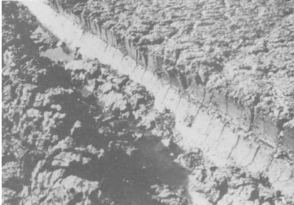
Figure 5-21. Closeup view of trenches formed by rotary trencher
