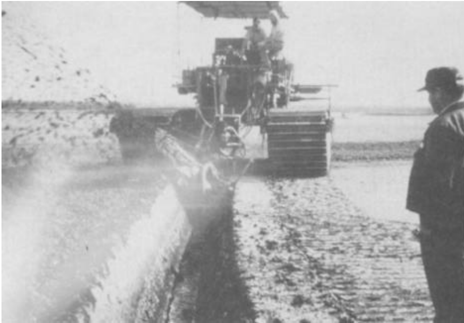
Figure 5-19. View of rotary trenching device in operation
