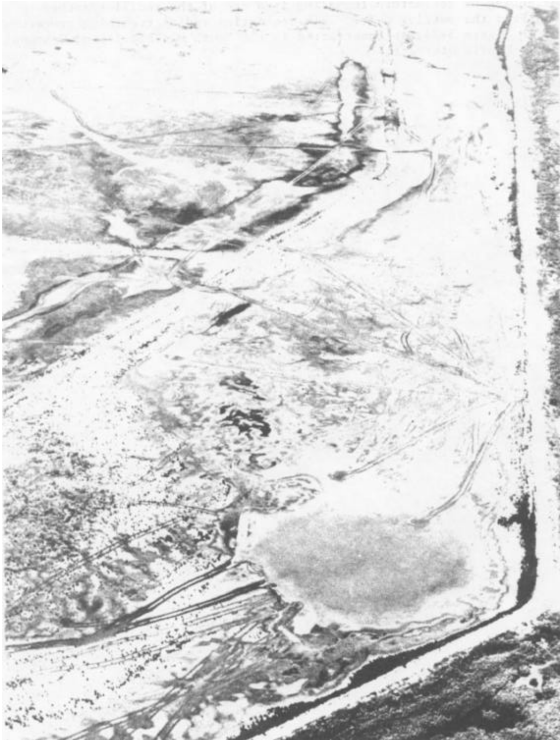
Figure 5-24. Aerial view of sequential radial trenching procedure used when interior cross dikes are encountered, South Blakely Island Disposal Site of the Mobile District
