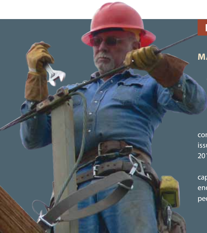
Lineman Ron Smith
