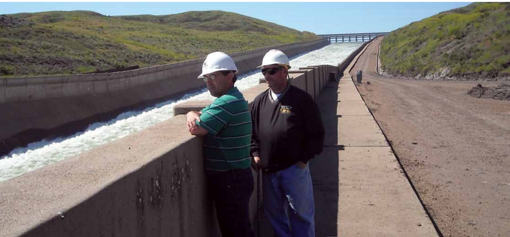
Safety and Occupational Health Specialists Scott McGaugh and Bruce Unger observe water flowing over the spillway at Fort Peck Dam.
