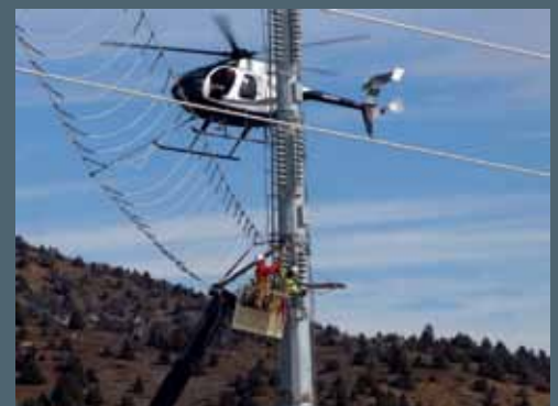
Western's line crews continued work on one of the Sacramento Voltage Support towers near Elverta, Calif., March 17, 2011. Because of the extremely wet conditions along the route, helicopters were used to transport workers, material and equipment to and from the towers.
