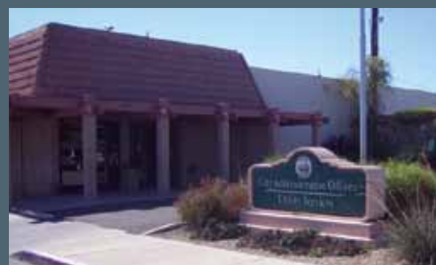
Needles’ Administrative building and utilities services
