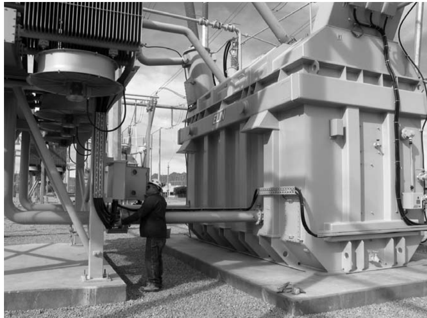
DSW Construction Representative Jim Jennings inspects the control cabinet of the 500/230-kV transformer (KT2A transformer bank) at the Mead Substation.
