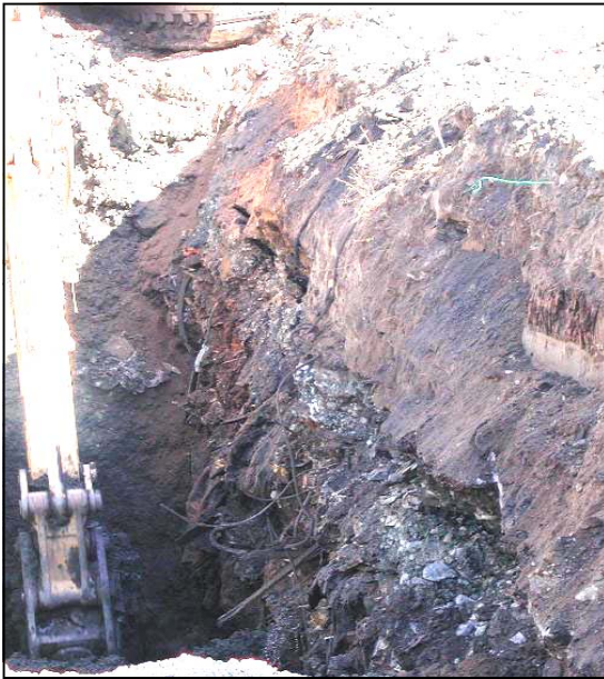
Typical Waste in Parcel E-2 Landfill. Note continuous layer of construction debris and trash that begins several feet below the ground surface.
