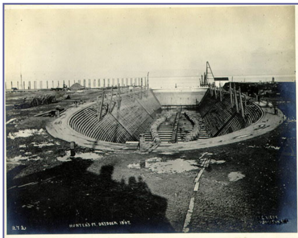
Original Drydock under Construction -- 1867
