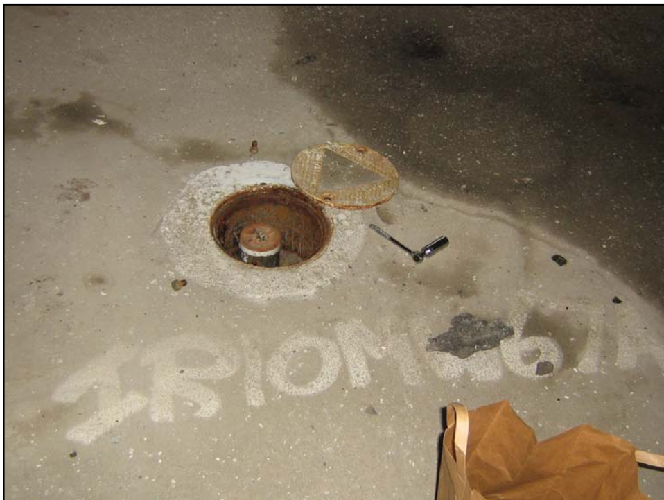
Well IR10MW67A; Well is in good condition, not locked, and there is no water in vault. Photo orientation - East Date 09 Jan 08
