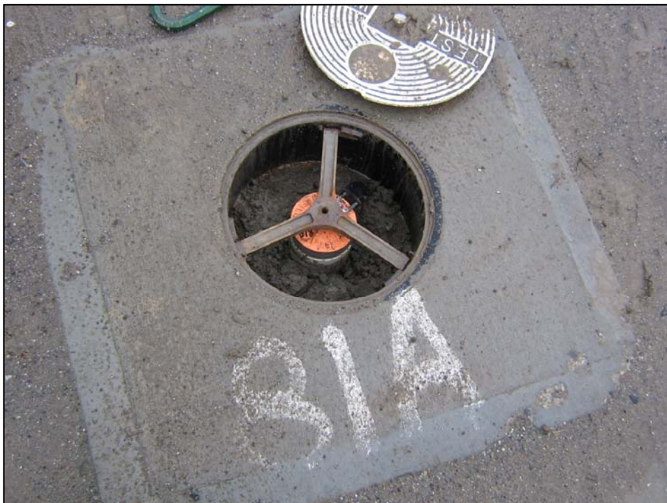
Well IR10MW81A; Well is in good condition, locked, and there is no water in vault. Photo orientation - West Date 10 Jan 08
