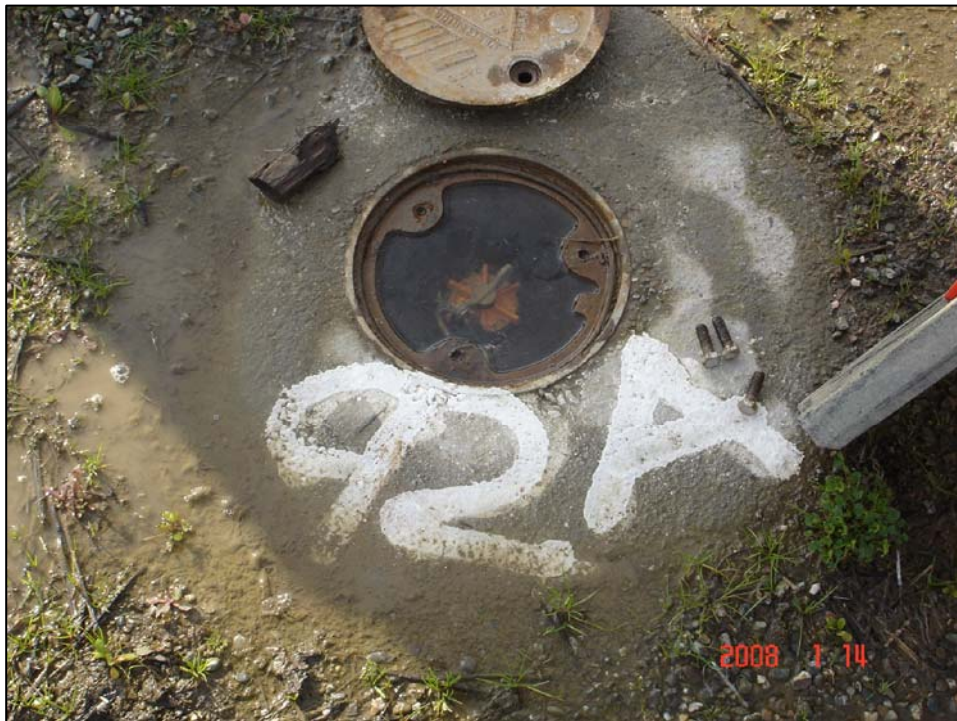
Well IR18MW92A; Well is in good condition, locked, and there is water in vault. Photo Orientation - West Date 14 Jan 08
