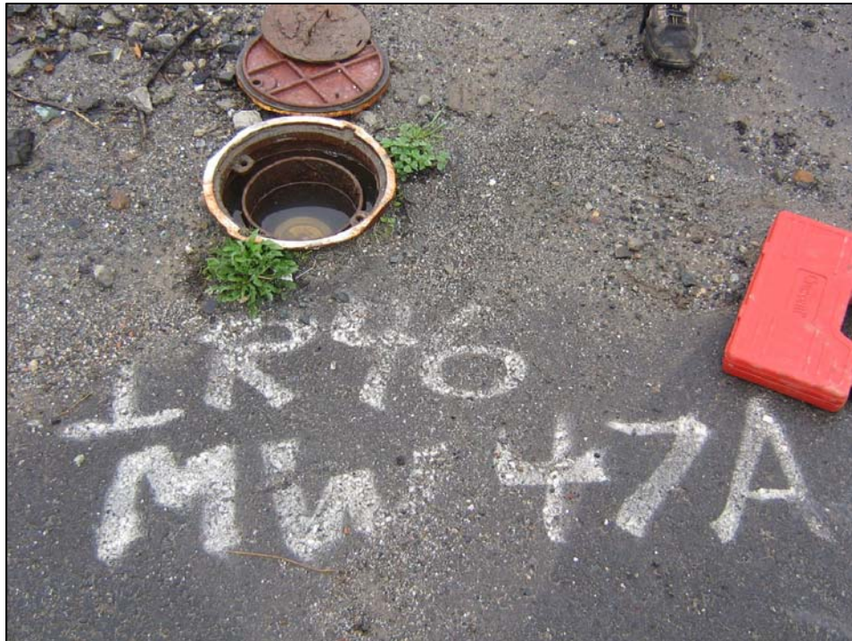
Well IR46MW47A; Well is in good condition with missing bolt, locked and there is water in vault. Photo orientation - North Date 10 Jan 08
