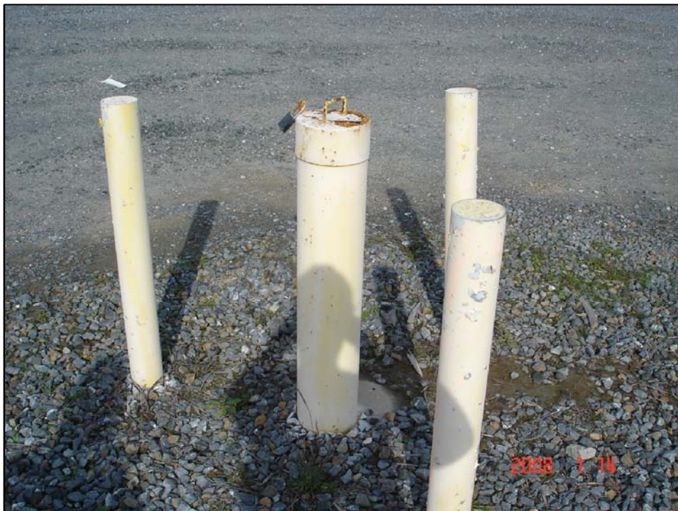
Well IR07MW26A; Well is in good condition, and locked. Photo Orientation - East Date 14 Jan 08
