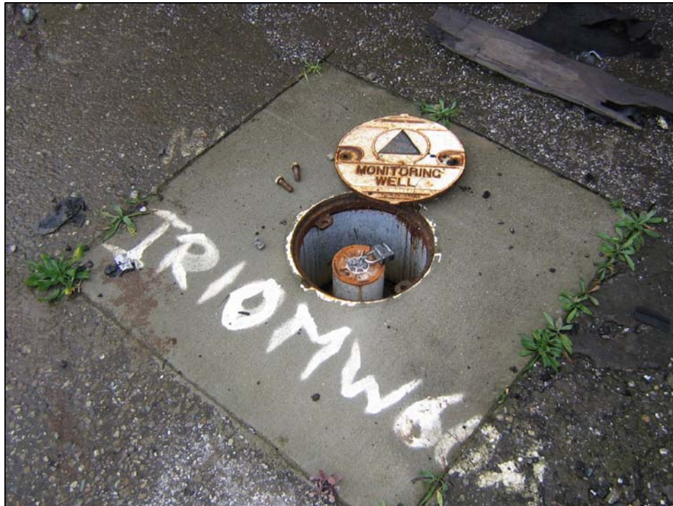
Well IR10MW60A; Well is in good condition, locked, and no water in vault. Photo Orientation South Date 09 Jan 08
