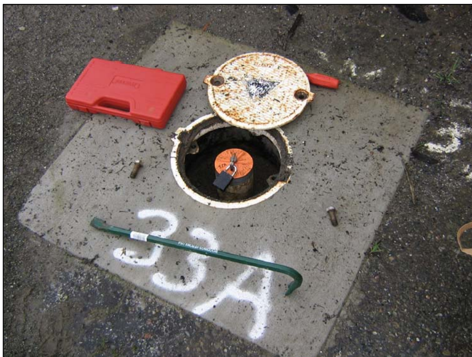
Well IR10MW33A; Well is in good condition and locked. Photo orientation - South Date 09 Jan 08
