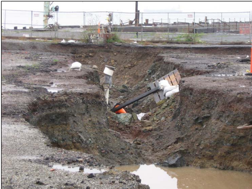
Well IR07MW19A; Well has been excavated. Photo orientation - East Date 09 Jan 08
