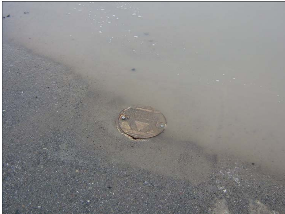
Well IR10MW80A; Well is under water. Photo orientation - North Date 10 Jan 08
