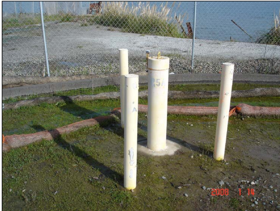
Well IR25MW25A; Well is in good condition, locked. Photo Orientation - East Date 14 Jan 08
