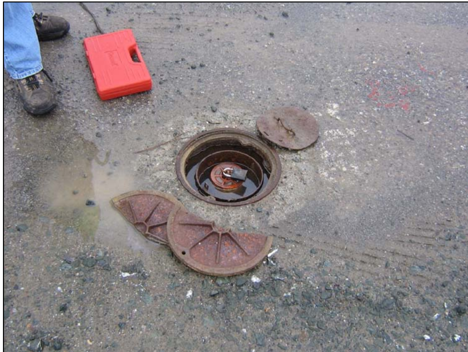
Well IR10MW32A; Well has cracked lid, locked, and water in vault. Photo orientation - West Date 10 Jan 08
