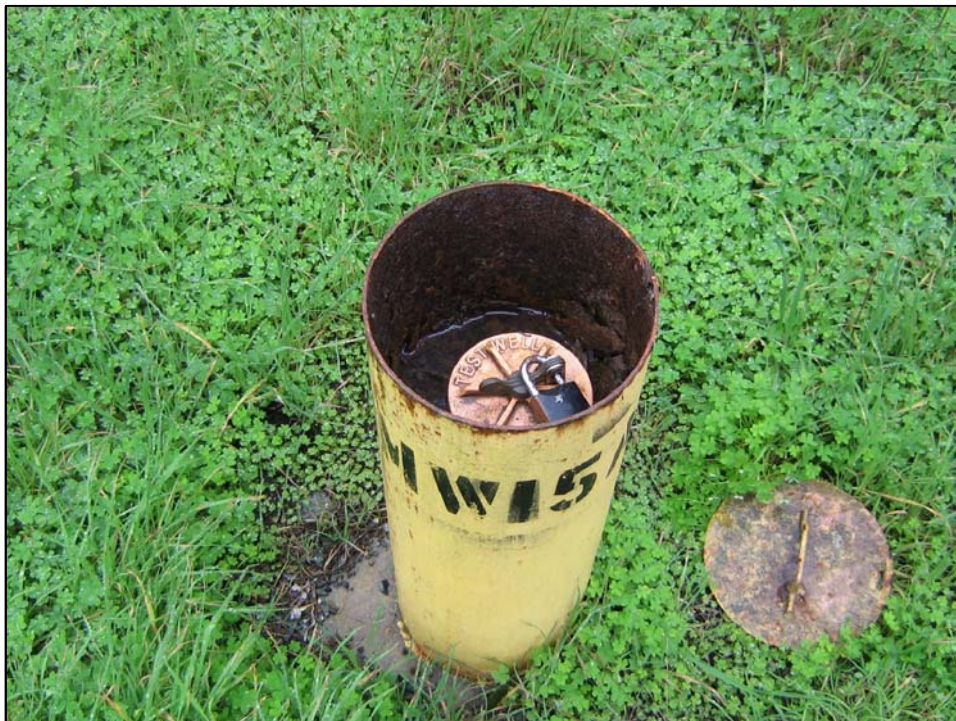
Well UT02MW15A; Well is in good condition, locked with small amount of water in vault. Photo orientation - South Date 10 Jan 08
