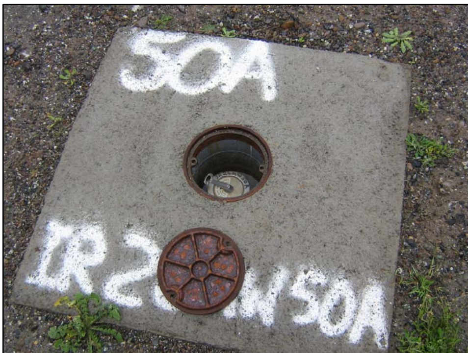
Well IR26MW50A; Well is in good condition, locked, and water in vault. Photo orientation - North Date 10 Jan 08
