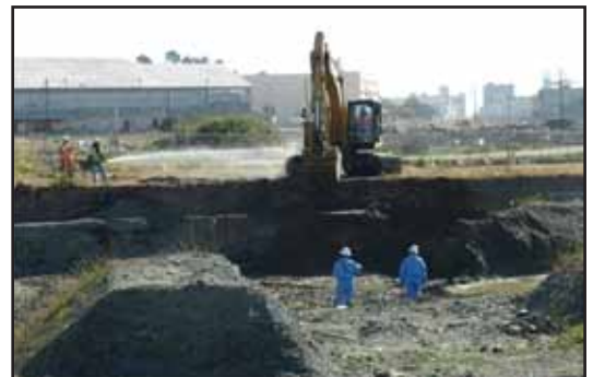
Excavation of soil with lead contamination
