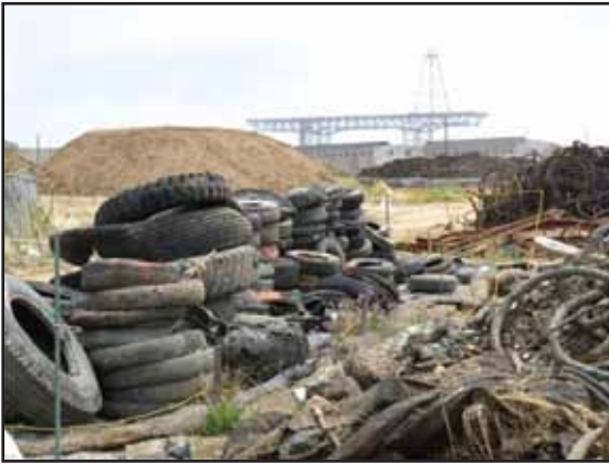
Debris excavated from PCB Hot Spot
