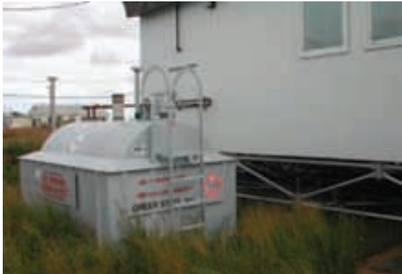
Napakiak ANG facility with a modern fuel storage tank. D. Rudis/USFWS photo
