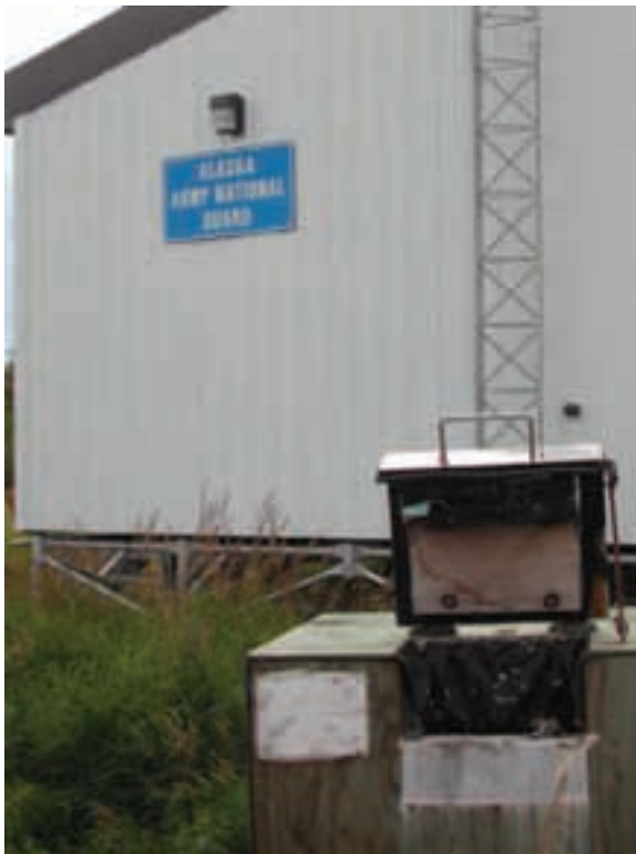
Napakiak community honey bucket dumping station located adjacent to the ANG site. D. Rudis/USFWS photo
