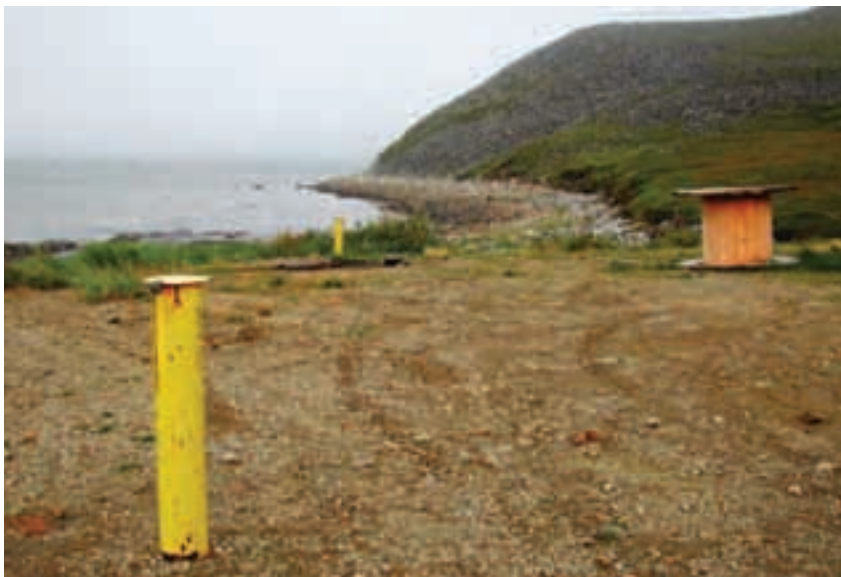
Cape Romanzof LRRS site landfills are graded and have closure signs. Those with surface and groundwater contamination have monitoring wells. D. Rudis/USFWS photo
