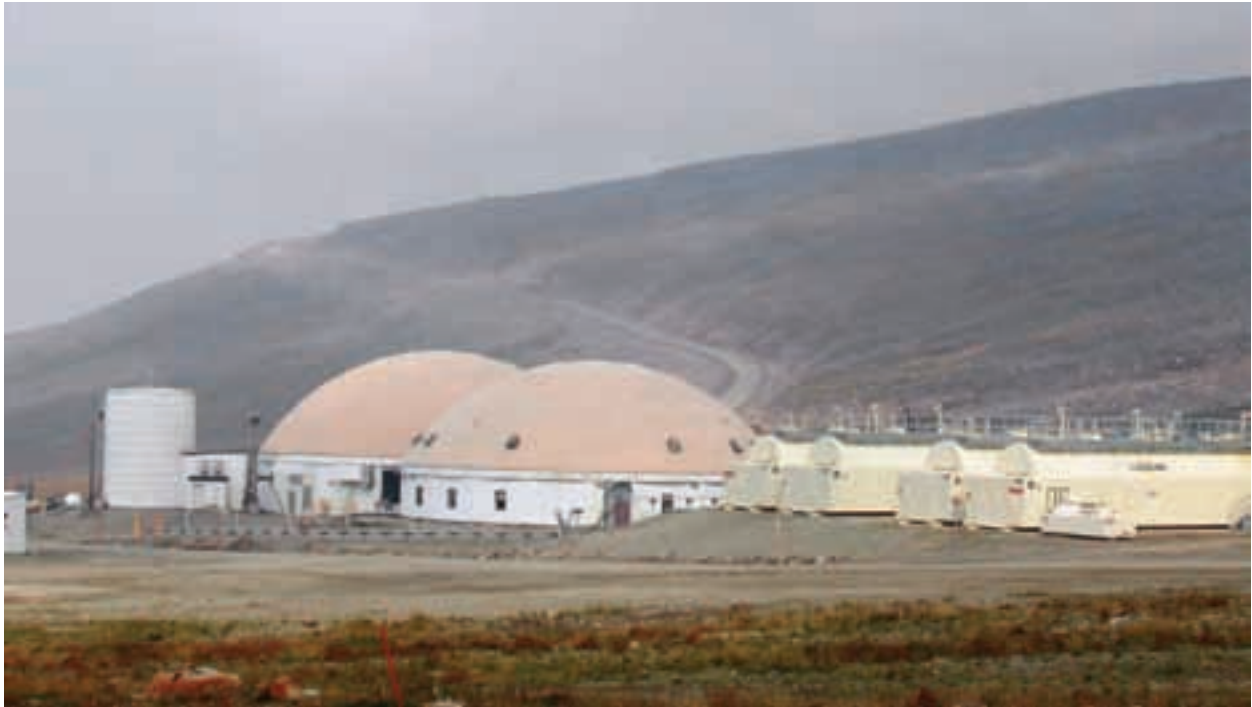
The Cape Romanzof LRRS base station and fuel storage area. This site has a history of fuel spills. D. Rudis/USFWS photo
