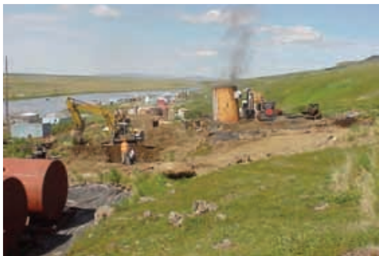
Thermal remediation was used to clean petroleum hydrocarbon contaminated soils at the Nightmute School site. Engineering/USFWS photo.
