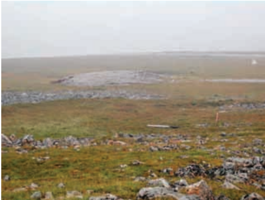
The 1992 Service study found that Landfill Number 2 (LF03) at the Cape Romanzof LRRS was a primary contributor of contaminants, including PAHs, PCBs, chlordane, lead, and cadmium to Fowler Creek sediments. D. Rudis/USFWS photo
