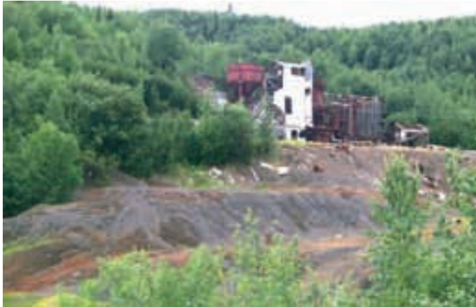
In early 2008, the U.S. Environmental Protection Agency reevaluated the Red Devil Mine, determining that the site's Hazard Ranking Score was high enough to make the mine site eligible for placement on the Superfund National Priorities List. BLM photo.
