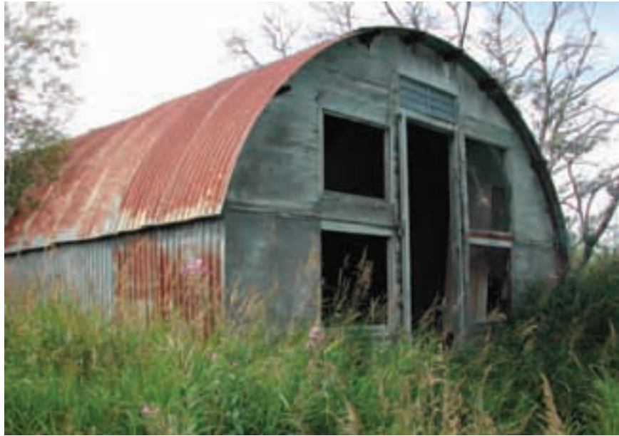
Todd Army Airfield quonset hut surrounded by vegetation. D. Rudis/USFWS photo
