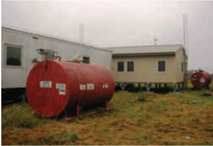
Alaska Army National Guard (ANG) building and fuel supply tank in Akiachak. Most villages in the refuge have similar ANG buildings and associated fuel tanks. D. Rudis/USFWS
