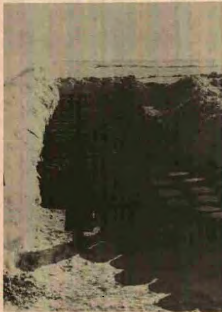
German fuel stores protected by snow revetments in Russia.
