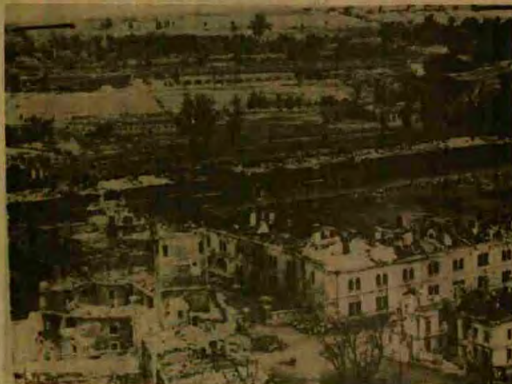
The citadel of Brest-Litovsk, showing heavy damage by the GAF, 1941
