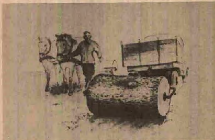
Improved rollers fashioned from tree trunks, used by the Russians in airfield construction
