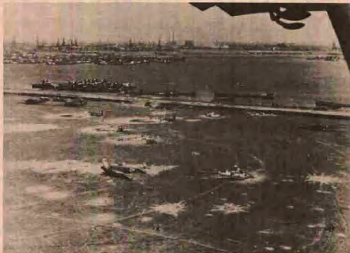
Destroyed Ju-52's at Waalhaven Airport; Rotterdam in the distance
