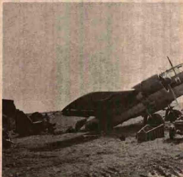
Figure 24 Damage caused by Soviet air attacks on the field at Smolensk-North
