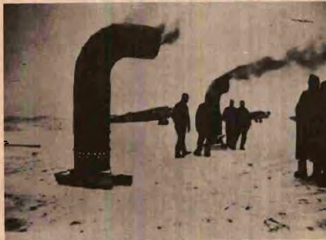
Figure 38 Provisional warming ovens for German aircraft engines in Russia, 1941
