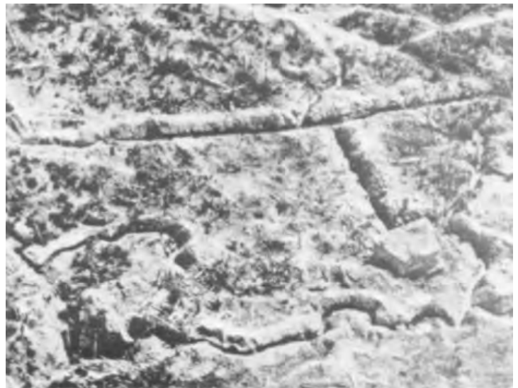
An aerial view of trenches taken during photo reconnaissance.
