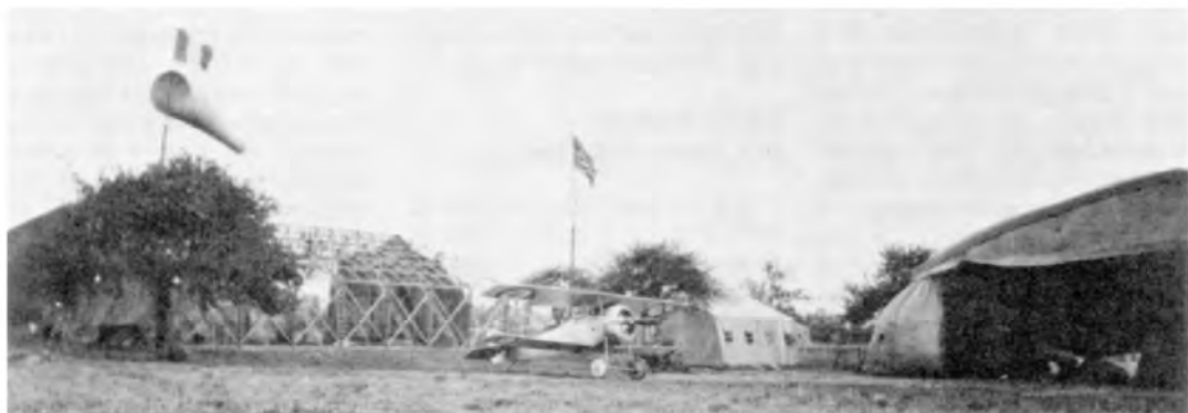
Lafayette Escadrille hangars at Ham airdrome.
