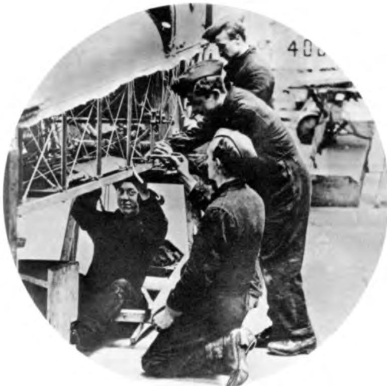
Aviators constantly trained to keep abreast of changing methods and technology in aerial warfare (above). Air Service recruits learn to wire a fuselage (right).
