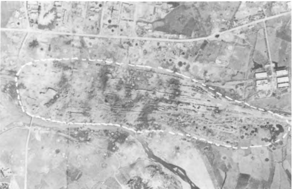
Rippled trackage, cratered railbeds, and damaged box and rail cars are evidence of the accuracy of B-29 attacks.
