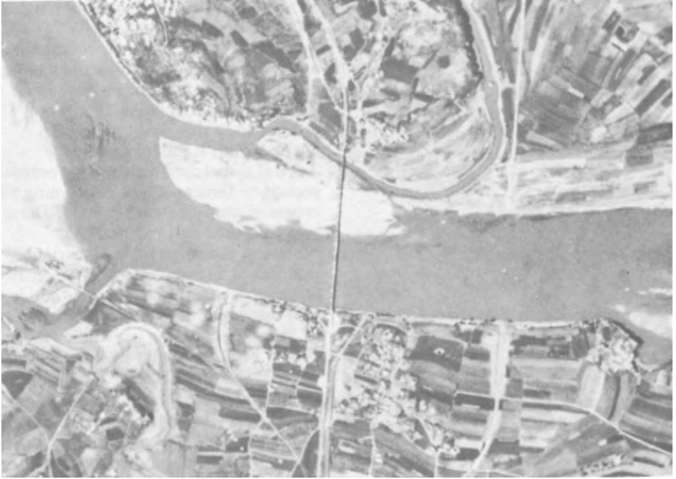
A rail bridge near Suncheon, North Korea before B-29's of the 98th Bomb Wing dropped it on 1 September.
