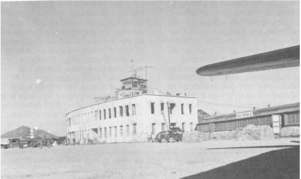
Base Operations and control tower, Kimpo AB.
