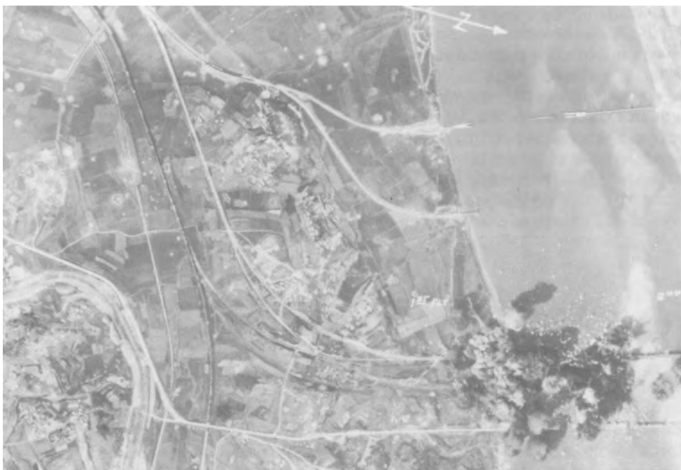
Five rail and highway bridges are knocked out at this rail complex near Sinanju, 4 September 1951.
