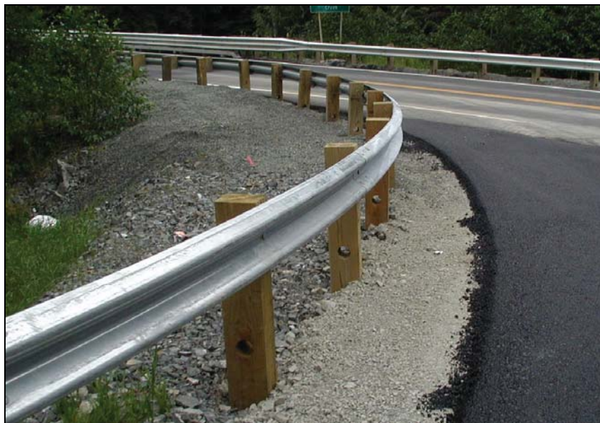
Figure 4.7: Curved Rail Guardrail
