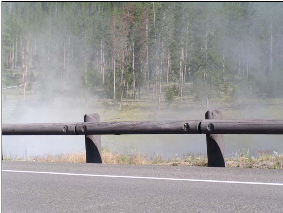
Figure 3.8: Steel-Backed Log Rail, SBL
