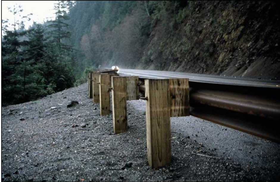
Figure 3.5: Strong Post W-Beam, G4
