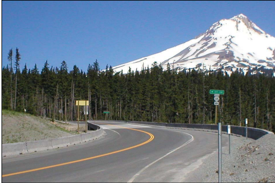
Figure 3.7: Concrete Safety Shape, CSS
