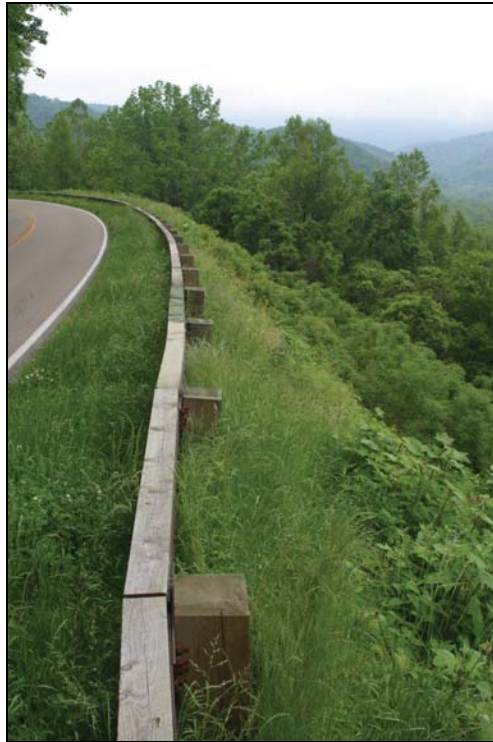
Figure 3.10: Precast Concrete Guardwall, PCG
