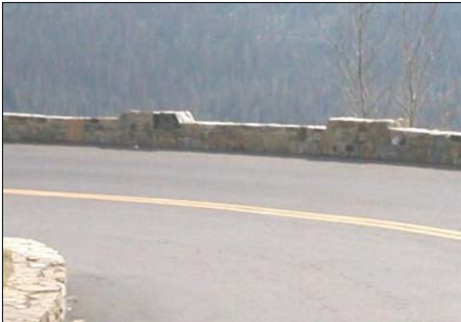
Figure 3.12: Random Rubble Cavity Wall, RCW
