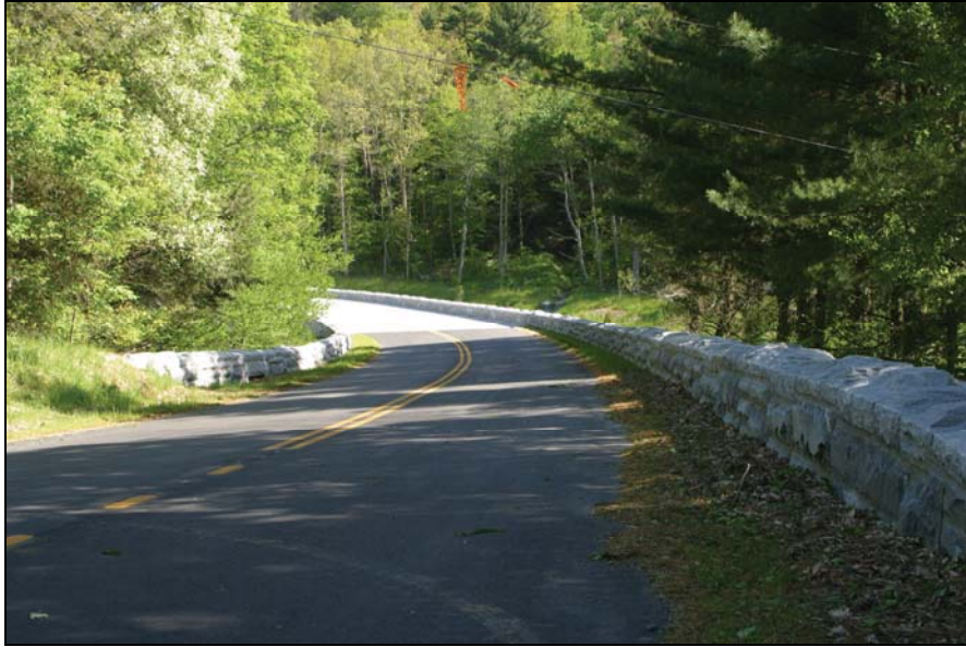
Figure 3.12: Random Rubble Cavity Wall, RCW
