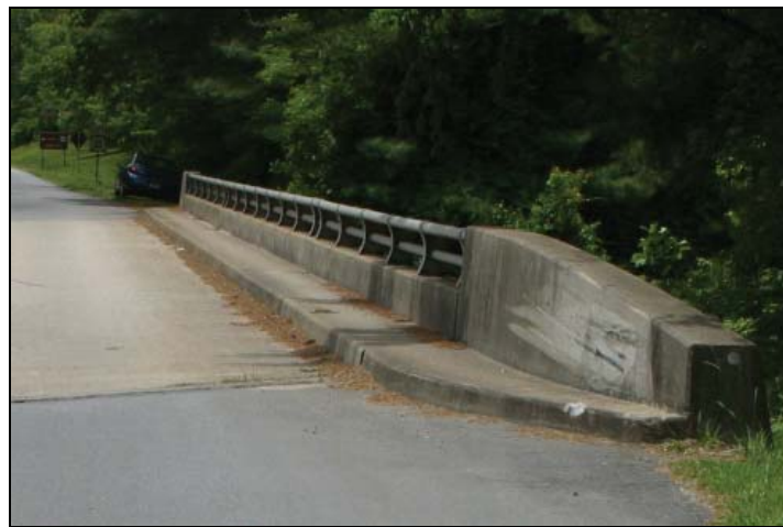
Figure 2.3: Unshielded Bridge Rail End
