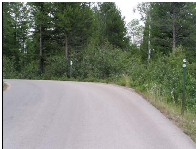
Figure 2.5: Delineation on a Horizontal Curve
