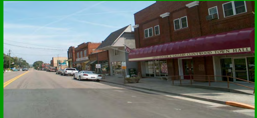
Store Fronts and Sidewalks
