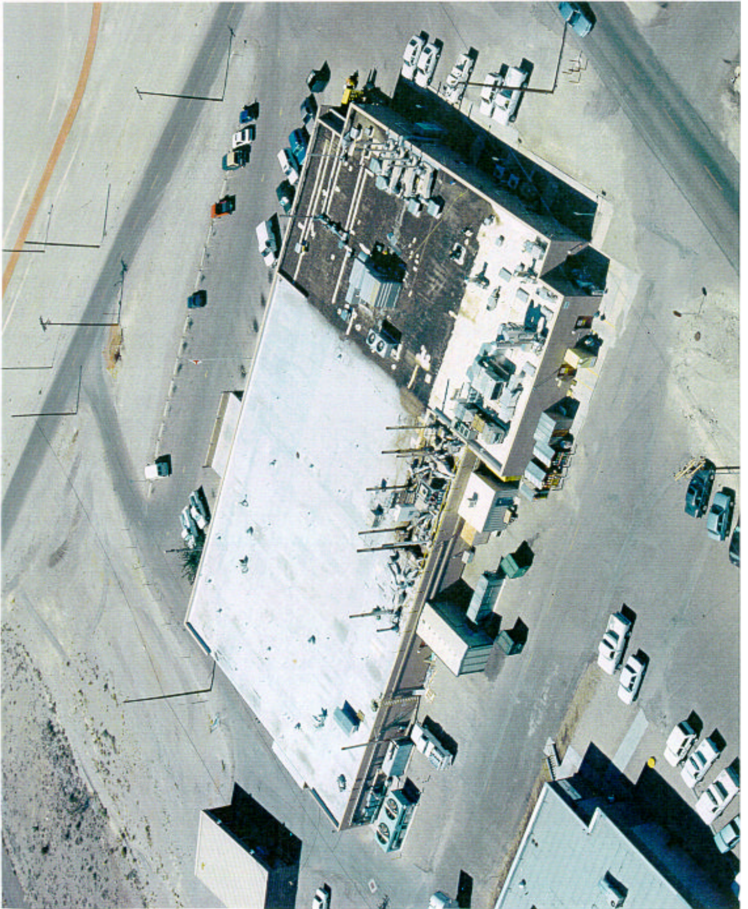
Figure 4.0 Photograph of the Building 650 Hood Ventilation Stacks Seen from Above (Photo Date Not Available)
