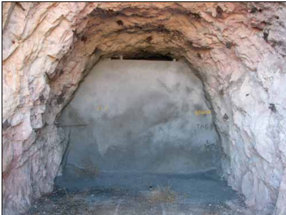
Figure 6-15. Bat-compatible closure at 16A Tunnel
