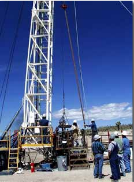
Workers install pump at a well
