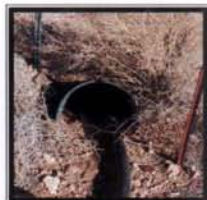
Burrow A Culvert Aspect: 270° (W) Height: 26 cm Width: 35 cm
