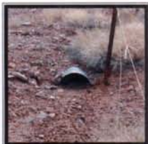
Burrow A Culvert Aspect: 20° (N) Height: 20 cm Width: 38 cm
