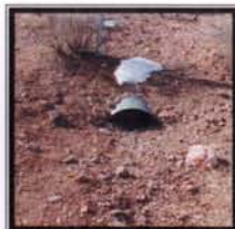
Burrow D Culvert Aspect: 60° (NE) Height: 15 cm Width: 32 cm
