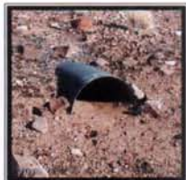
Burrow A Culvert Aspect: 260° (W) Height: 21 cm Width: 38 cm
