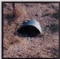
Burrow A Culvert Aspect: 350° (NE) Height: 15 cm Width: 36 cm
