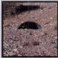
Burrow B Culvert Aspect: 180° (S) Height: 17 cm Width: 37 cm
