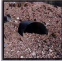
Burrow H Culvert Aspect: 50° (NE) Height: 28 cm Width: 34 cm
