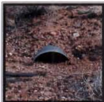
Burrow B Culvert Aspect: 270° (W) Height: 12 cm Width: 32 cm
