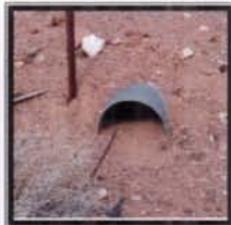
Burrow C Culvert Aspect: 200° (S) Height: 23 cm Width: 35 cm
