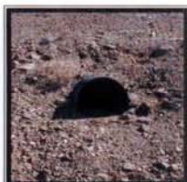
Burrow A Culvert Aspect: 340° (NE) Height: 27 cm Width: 39 cm
