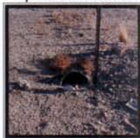
Burrow A Culvert Aspect: 330° (NW) Height: 20 cm Width: 35 cm
