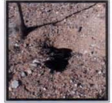
Burrow E Culvert (Filled In) Aspect: 190° (S) Height: 8 cm Width: 16 cm
