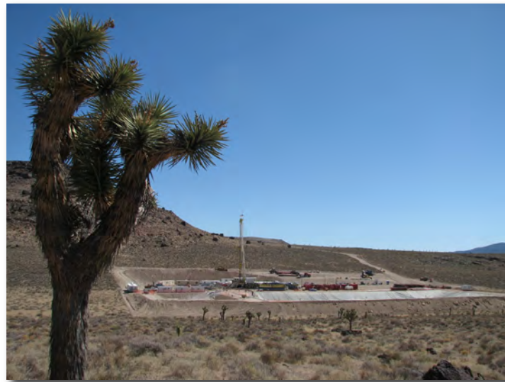
Well ER-EC-11 During Drilling
