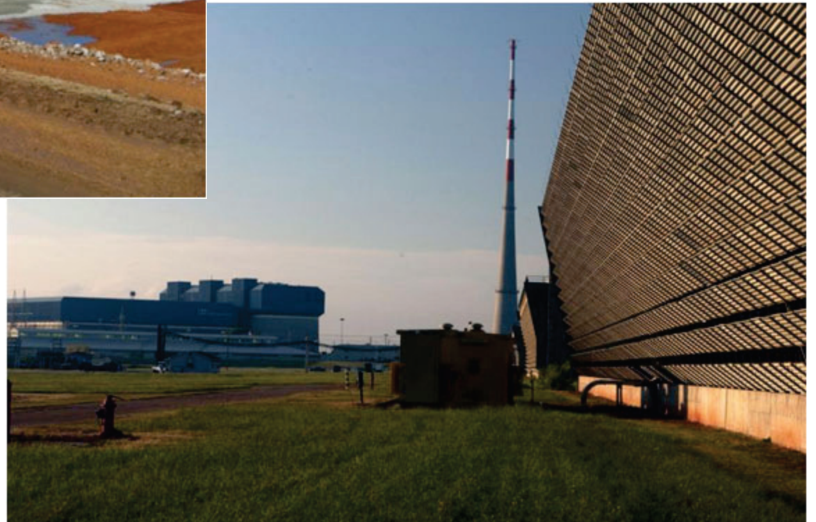
Existing Cooling Tower
