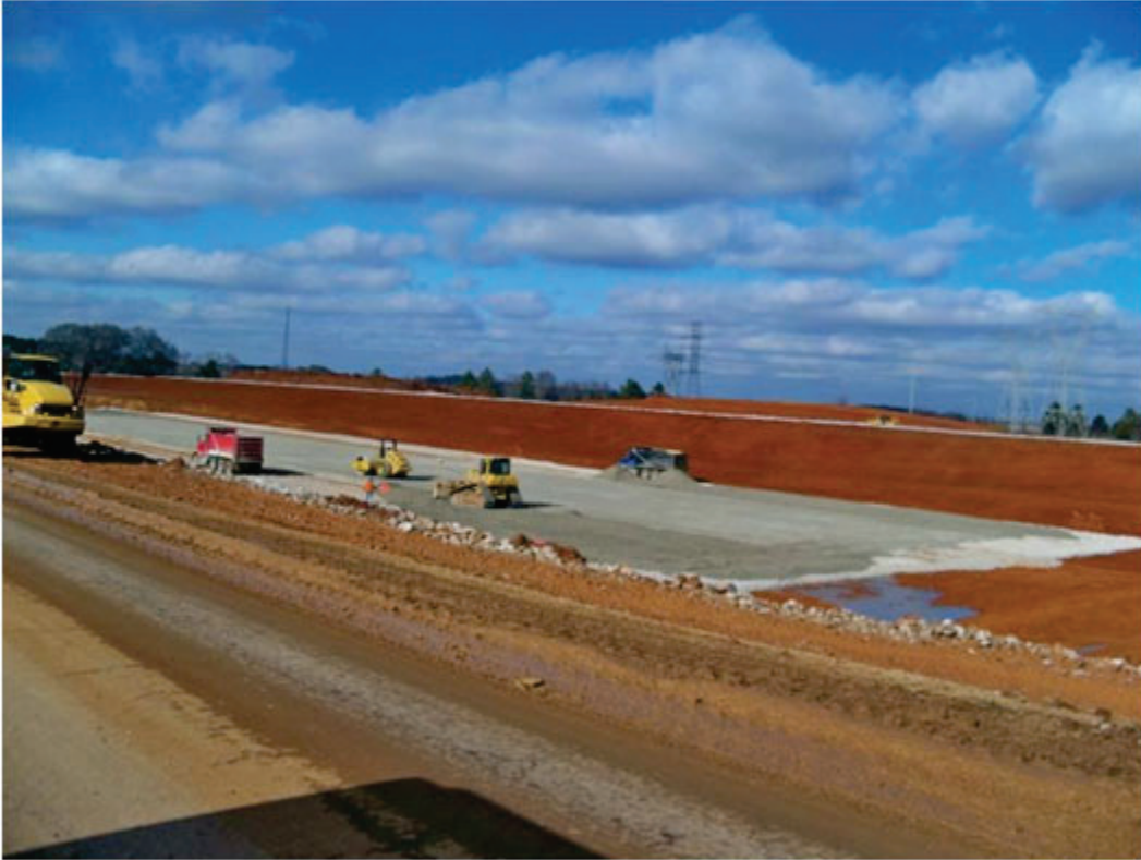
Grading for New Tower
