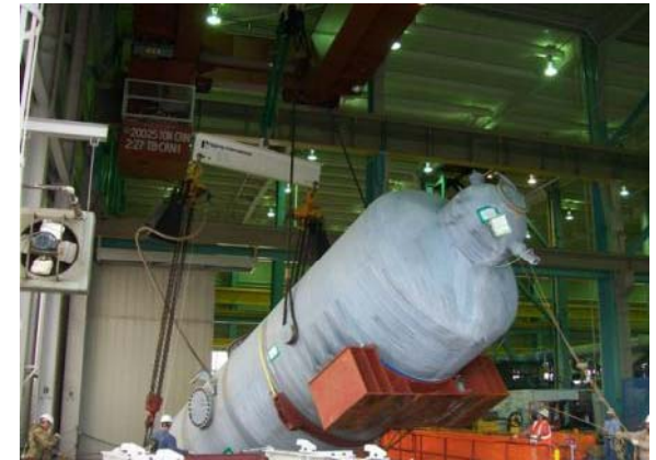
Moisture Separator Reheaters Installation in the Turbine Building
