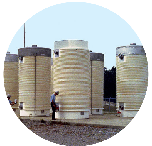
Currently, spent nuclear fuel is stored onsite at nuclear power plants, first submerged for months in pools to cool, then above ground in large casks.
