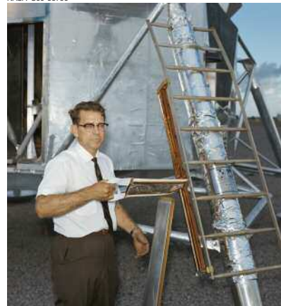
On a mock-up of the Lunar Module, David McCraw demonstrates the deployment sequence of the flag, following step-by-step procedures created for the astronauts. The entire flag unit fit into a three-foot protective heat shroud, stored on the side of the descent stage ladder.
