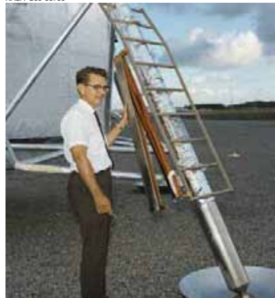
On a mock-up of the Lunar Module, David McCraw demonstrates the deployment sequence of the flag, following step-by-step procedures created for the astronauts. The entire flag unit fit into a three-foot protective heat shroud, stored on the side of the descent stage ladder.
