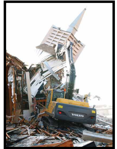
Demolition of the Eielson AFB Chapel
