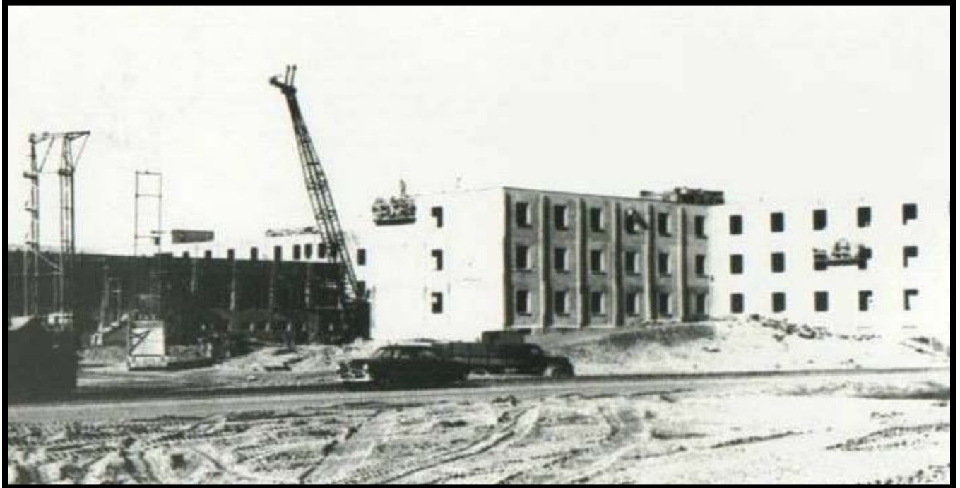
750-man barracks under construction (Amber Hall)
