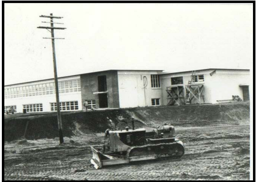
Pennell Elementary under construction
