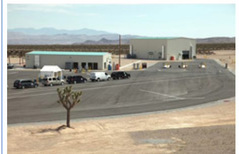
RNCTEC, hosting its first test campaign, Eland, in July-August 2009. The completed TSB is behind the cars on the left, with the portals on the right and the
