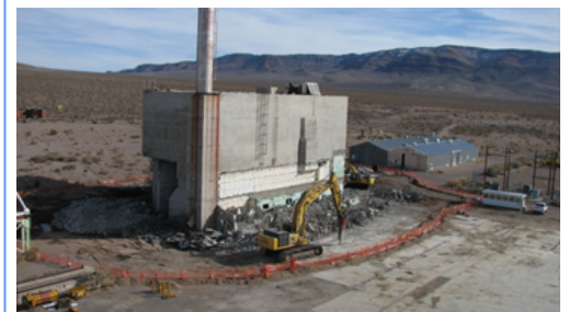
Demolition progress at the R-MAD Facility, December 2009.
