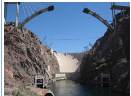
The Hoover Dam and by-pass bridge (under construction)
