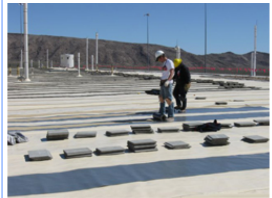
Workers renovate the roof of the DAF.
