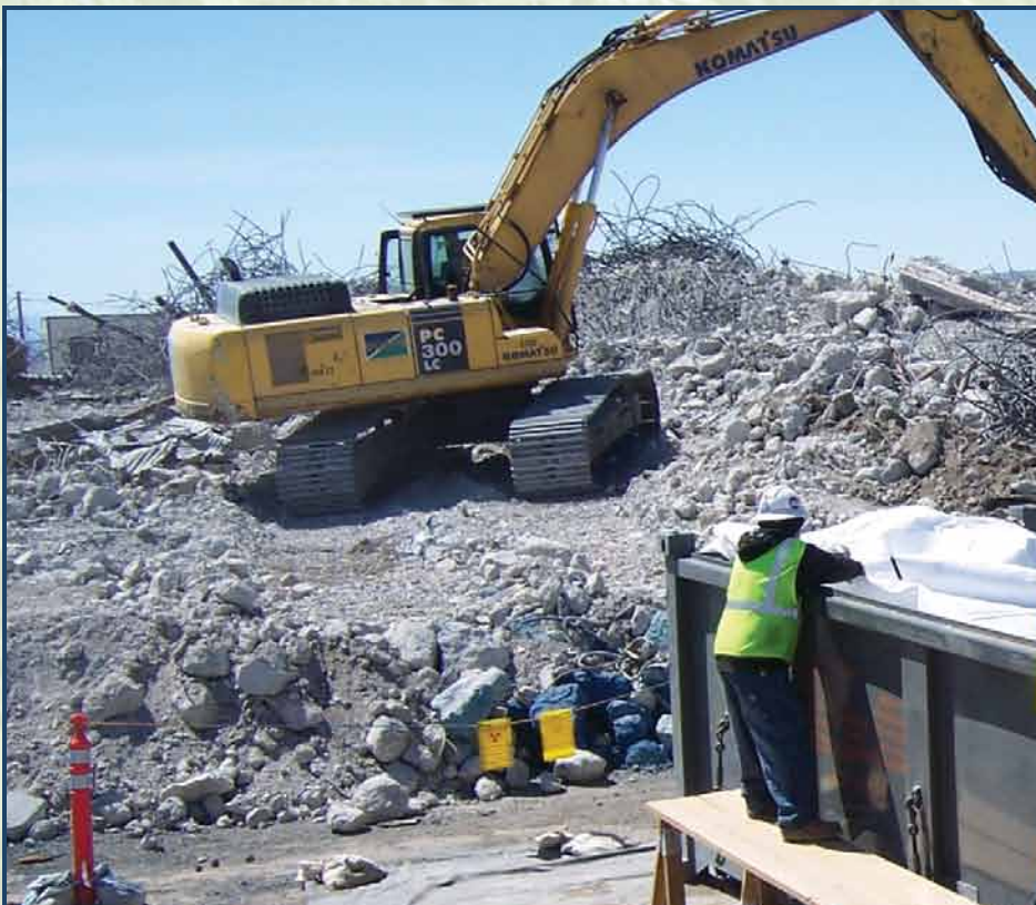
Low-level radioactive waste debris generated during R-MAD demolition is packaged for disposal at the NNSS Area 5 Radioactive Waste Management Site.
