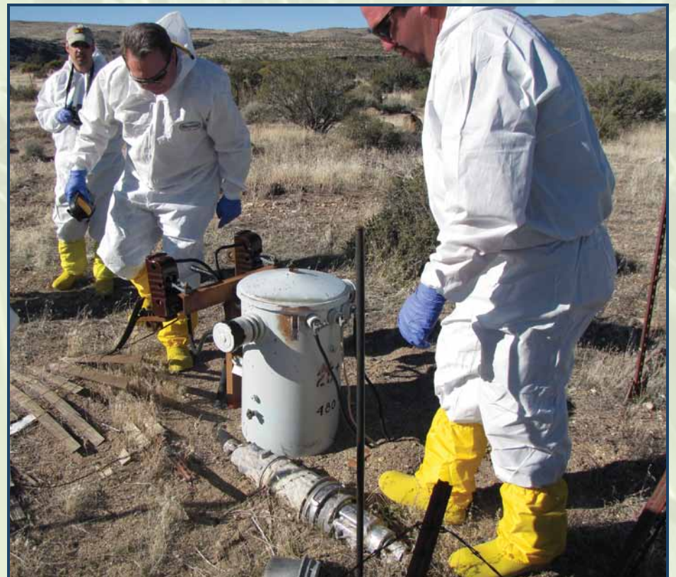
Workers examine an abandoned transformer at the BUGGY site in preparation for removal and disposal at the NNSS Area 5 Radioactive Waste Management Site as mixed low-level radioactive waste.
