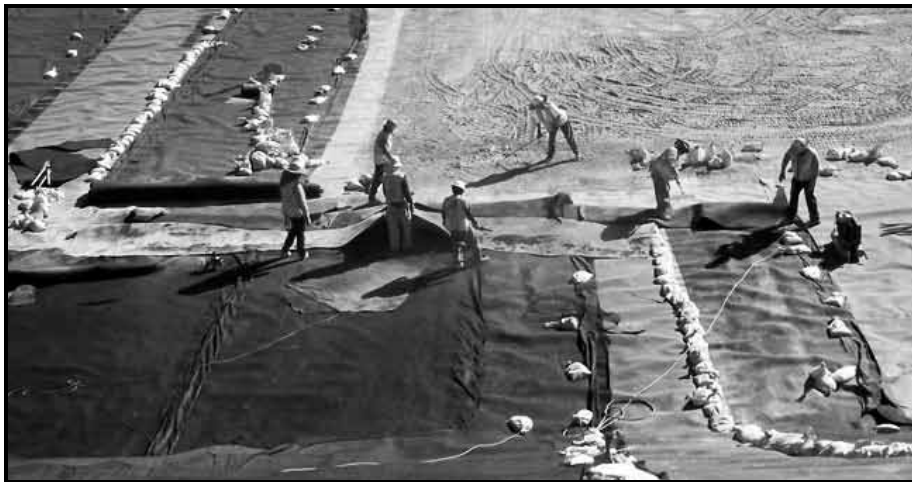
During construction, workers lined the unit with a five-layer geoliner.
