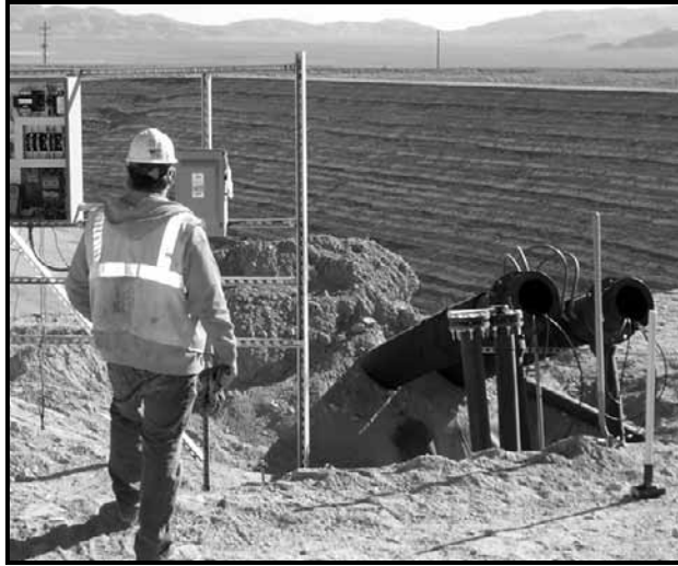
Workers test the leachate collection system.
