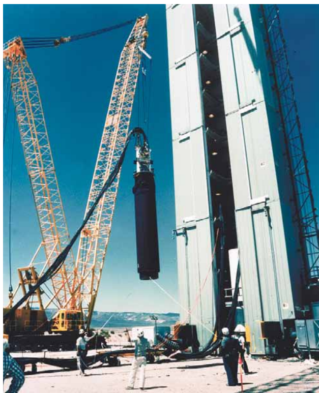
Workers prepare the Divider underground test (1992).
