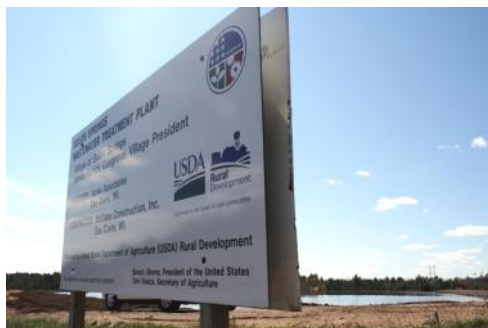
New lagoon and project sign for the Solon Springs Water Treatment Facility improvement and expansion project.
