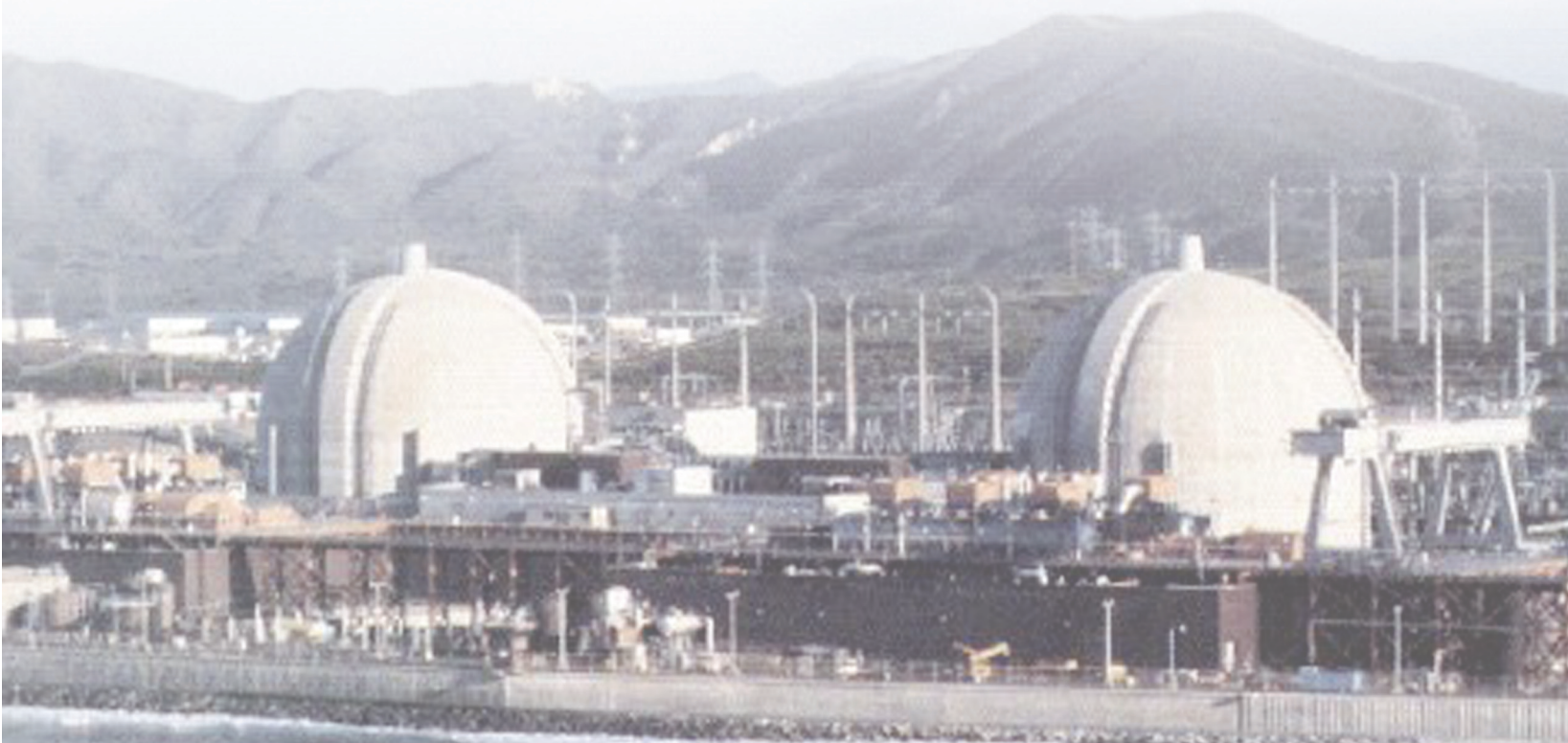
San Onofre Nuclear Generating Station in San Clemente, California.
