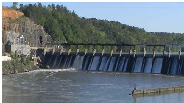
Figure 1. Bankhead Spillway at the Bankhead Lock and Dam in Tuscaloosa, Alabama
