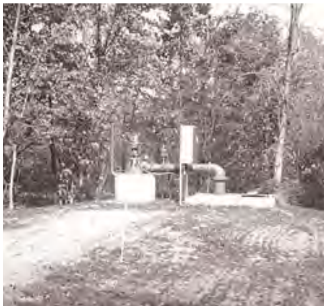
Public water supply well.
