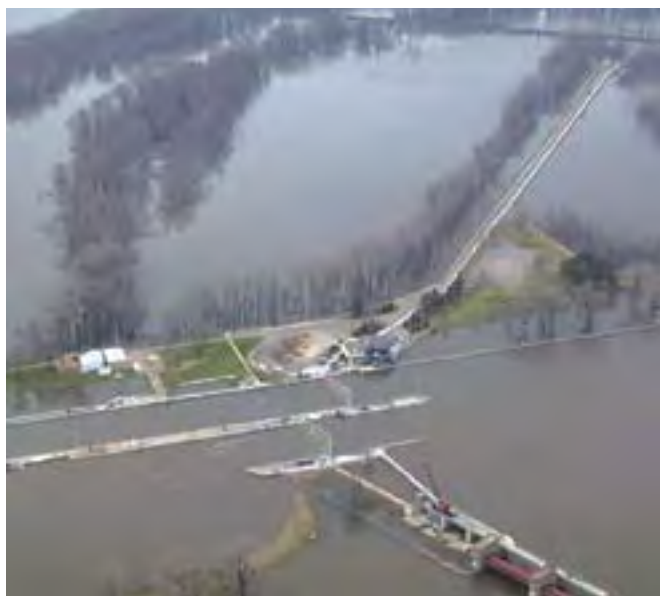
2001 Mississippi River flood: Locks and dam 5NM Northwest of Red Wing, MN along the Mississippi River. Photo by NOAA.
