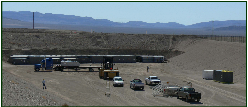
Mixed low-level radioactive waste disposal activities in the Pit 3 Mixed Waste Disposal Unit currently used at the Nevada Test Site Area 5 Radioactive Waste Management Site
