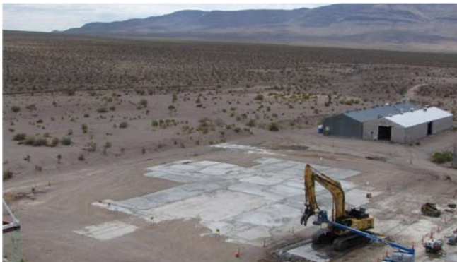
Work crews remove final remnants of demolished R-MAD facility in July.
