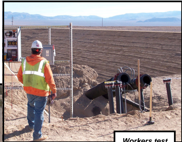
Workers test the leachate collection system.
