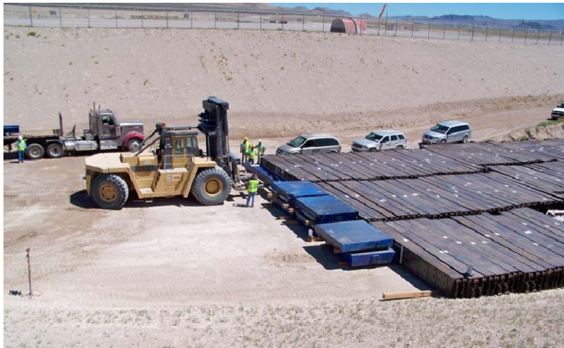
Seventeen percent of the Recovery Act waste disposed at the Area 5 RWMS was generated by cleanup activities on the Nevada Test Site. The waste seen here consists of beams and doors from dismantled nuclear rocket development facilities.
