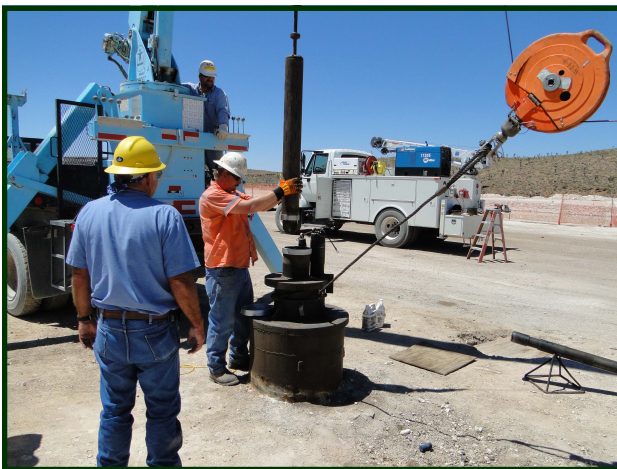
Field workers prepare to take down-hole measurements of a well.
